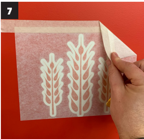
7 Peel / remove application mask. Go slowly. Be careful as the decal may peel away from surface.
